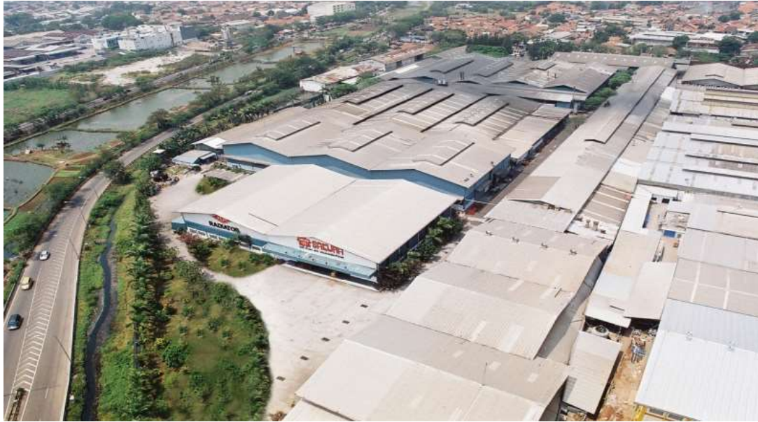
Kapuk Plant (Radiator Facilities)
